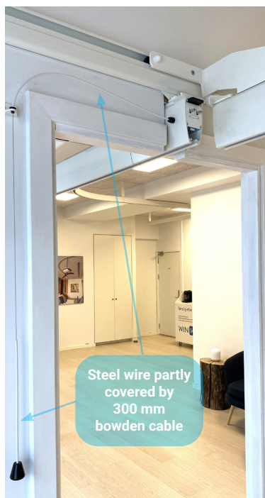
Pull the steel wire cord to activate and unlock the door connector. See step-by-step guide on next page.
